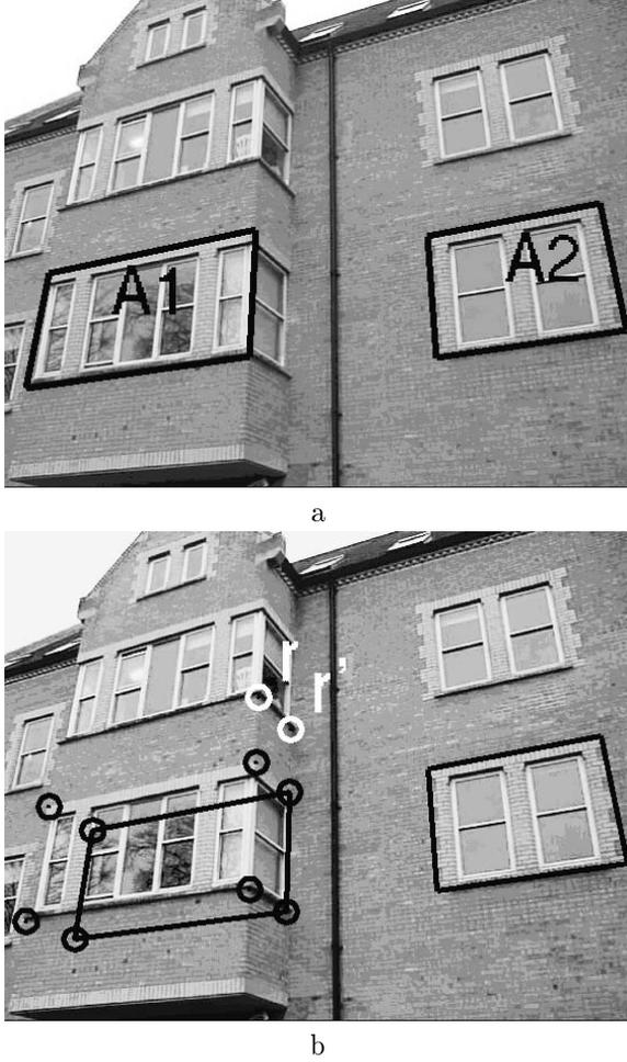
*Fig. 13. Measuring ratios of areas on separate planes:* (a) original image with two windows highlighted; (b) the left window is transferred onto the plane identified by  $\mathbf{r}'$  by the homology mapping (16). The two areas now lie on the same plane and can, therefore, be compared. The ratio between the areas of the two windows is then computed as:  $\frac{A_1}{A_2} = 1.45$ .
