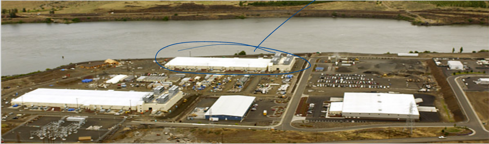
Google data centers in The Dalles, Oregon
