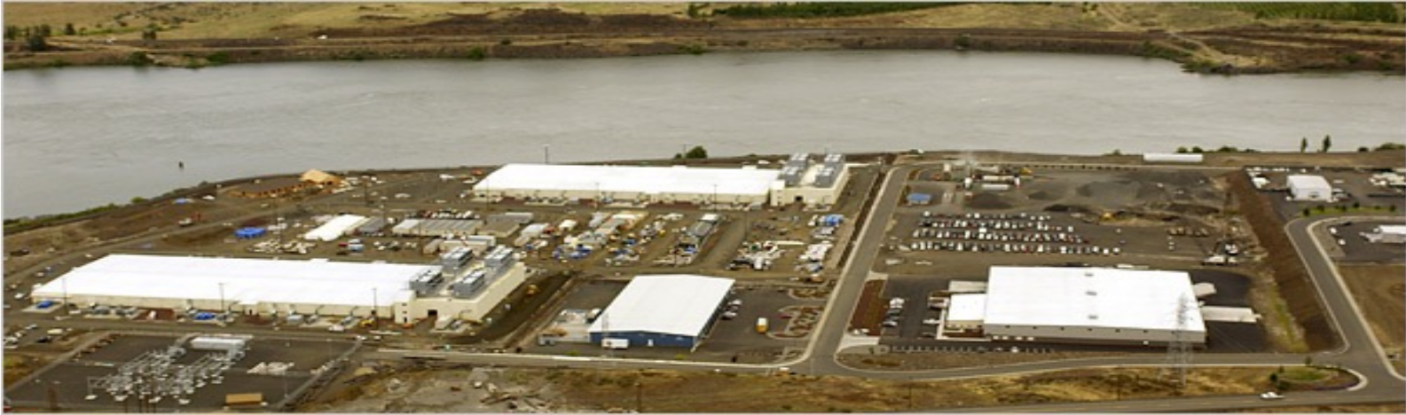
Google data centers in The Dalles, Oregon
