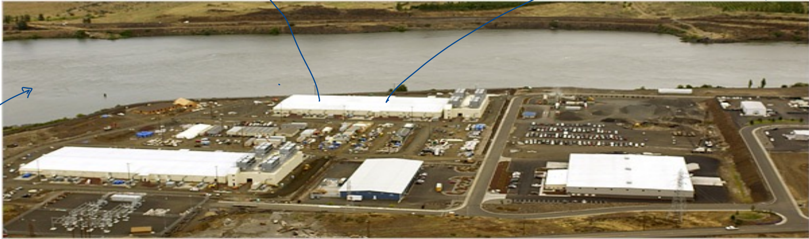
Google data centers in The Dalles, Oregon
