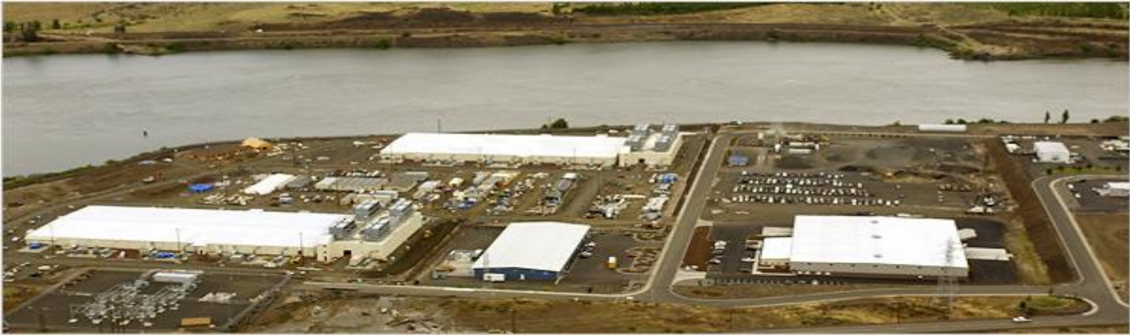
Google data centers in The Dalles, Oregon
