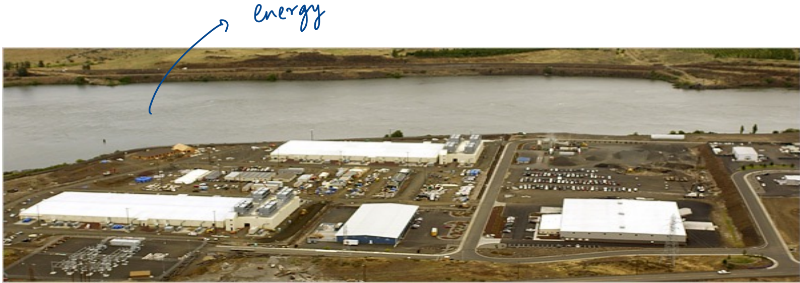
Google data centers in The Dalles, Oregon
